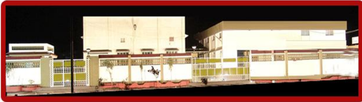
Ayushi Engineering Company - Front view
